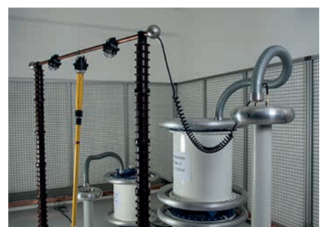
High voltage laboratory
