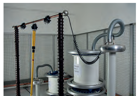
High voltage laboratory
